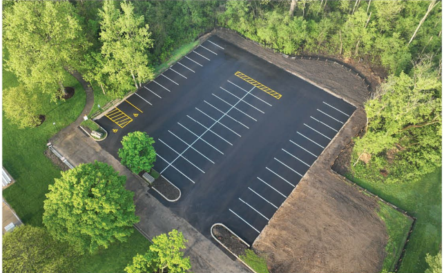
Waveland Park Parking Lot Expansion Completed May 2022
